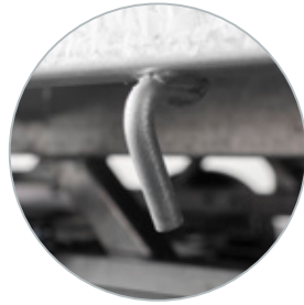
Long tie-hooks under the floor
